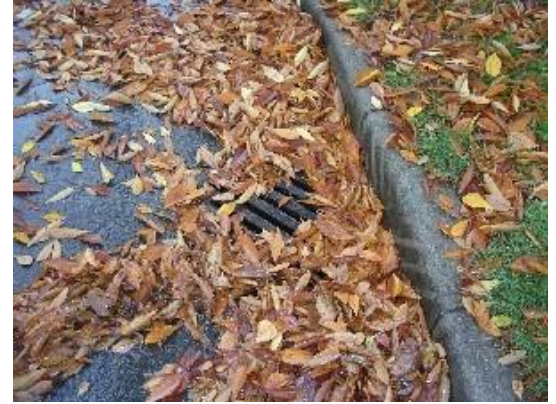
Clogged storm drains can lead to destructive flooding of streets and homes!
